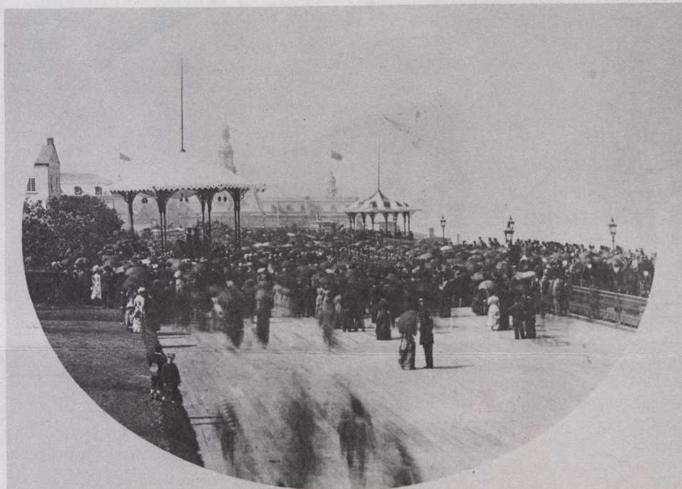
Inauguration of the Dufferin Terrace Quebec, 1879.
