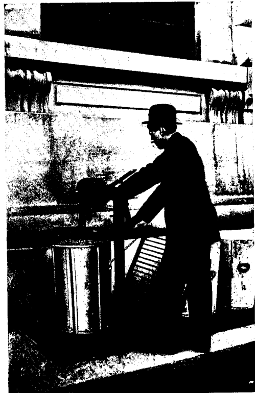
Hoist in Operation.
