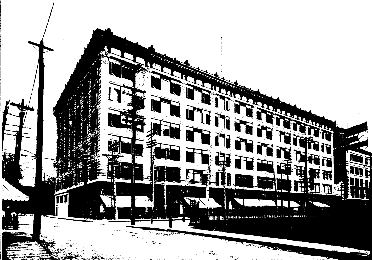
Jacobs Building, Montreal. Equipped with "Standard Ideal Ware." Mitchell & Creighton, Architects. W. J. McGuire, Plumber.
