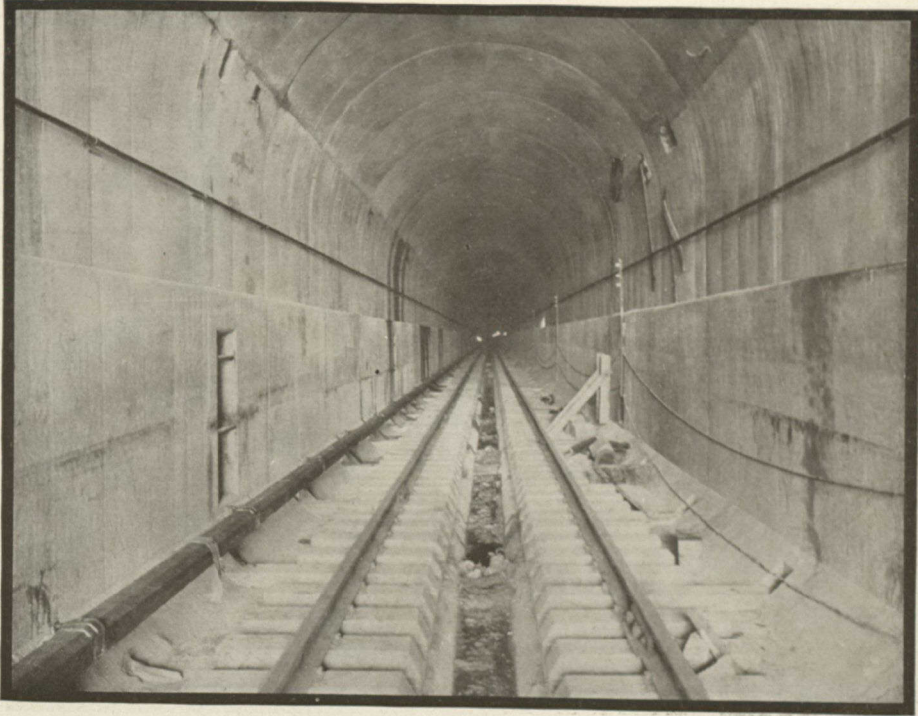
THE EASTBOUND TUBE FROM NEAR THE PORTAL ON THE WINDSOR SIDE.
