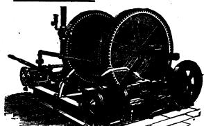
Double Cylinder Reversible Mine Engine.
