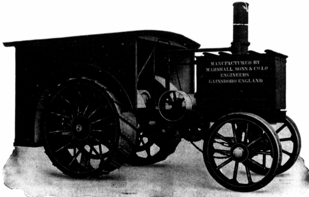
The above shows a 32 H.P. Draw Bar and 60-70 Brake H.P. Tractor. One Speed.
