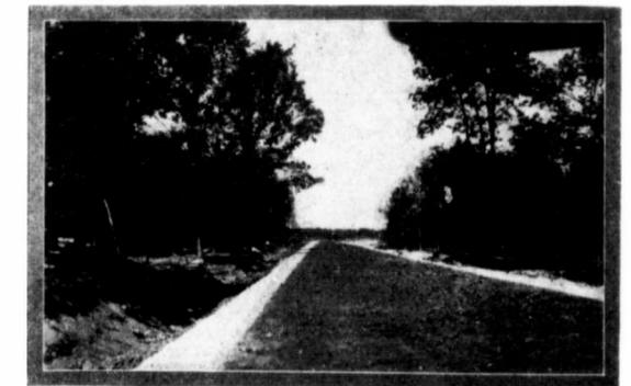
Road Completed and covered with Layer of Dirt to keep Moist while Setting
