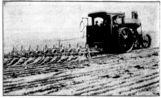
Avery Undermounted Steam Engine and "Self-Lift" Plow.
