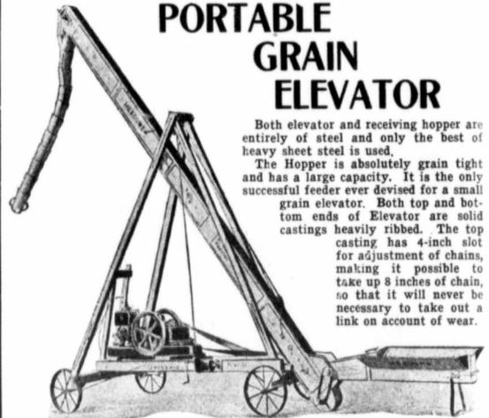
Both elevator and receiving hopper are entirely of steel and only the best of heavy sheet steel is used. The Hopper is absolutely grain tight and has a large capacity. It is the only successful feeder ever devised for a small grain elevator. Both top and bottom ends of Elevator are solid castings heavily ribbed. The top casting has 4-inch slot for adjustment of chains, making it possible to take up 8 inches of chain, so that it will never be necessary to take out a link on account of wear.
