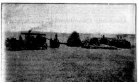
Threshing with an Avery Single Cylinder Steam Engine and "Yellow Fellow-Grain Saver" Separator.
