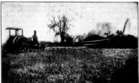
Threshing with an Avery Gas or Oil Tractor and "Yellow Fellow-Grain Saver" Separator.
