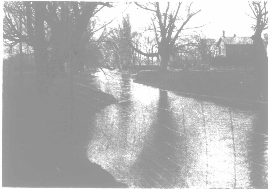
Mr. Haines' House, Meadowvale, Ont. Approach to Front Door.
