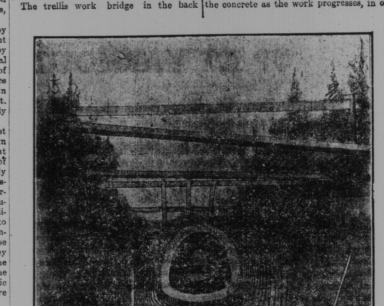
In the Trench Section of the Reinforced Concrete Pipe in Position
