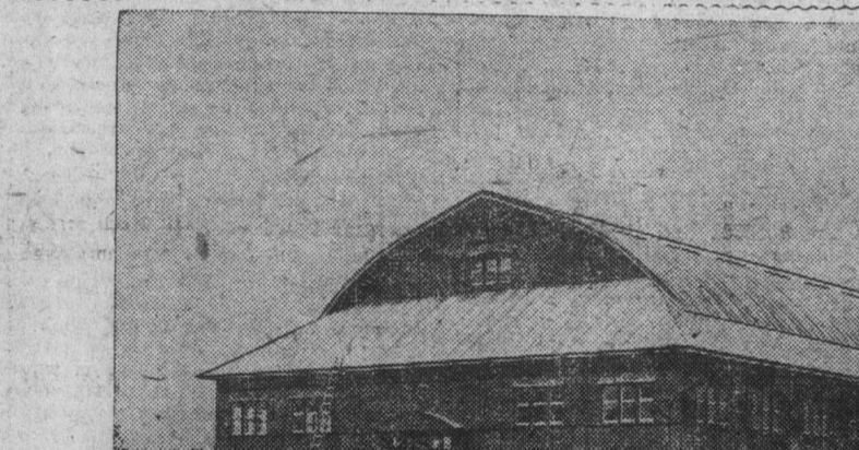
VICTORIA FAIR—MAIN BUILDING.
