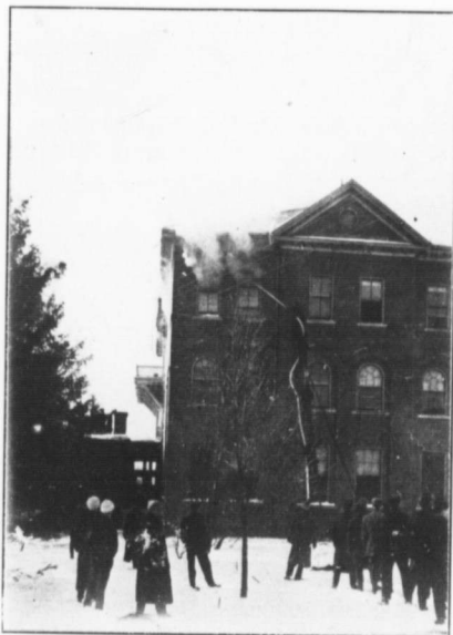
THE FIRE—THE BIOLOGY BUILDING BURNING.
