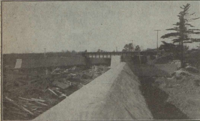
CANAL ENTRANCE AND SPILLWAY
