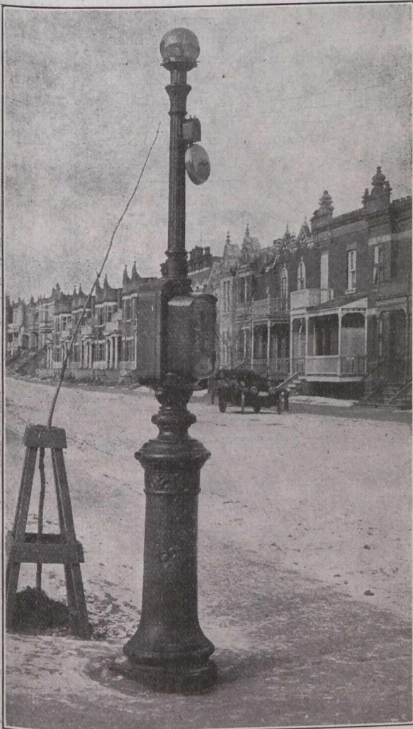
Police Signal Box and Flashlight Equipment, Mounted on Street Pedestal.
