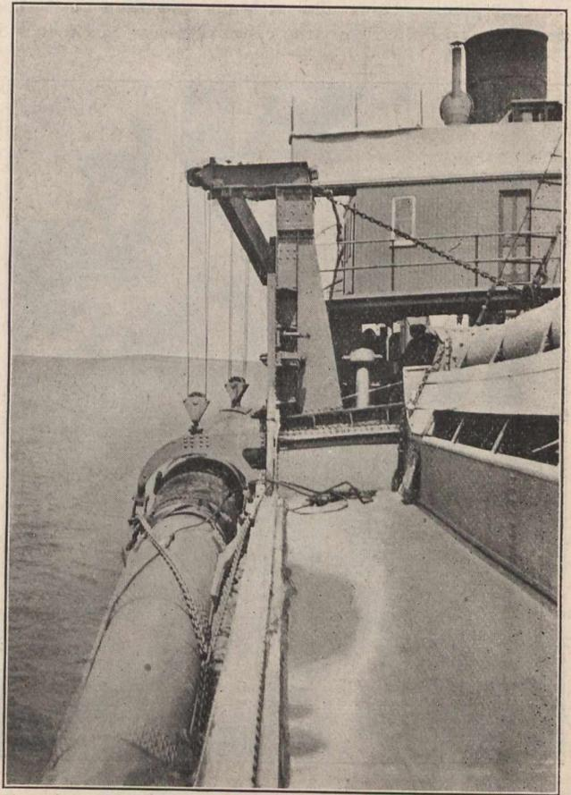
Fig. 4.—Suction Pipe partly submerged, showing leather joint.
