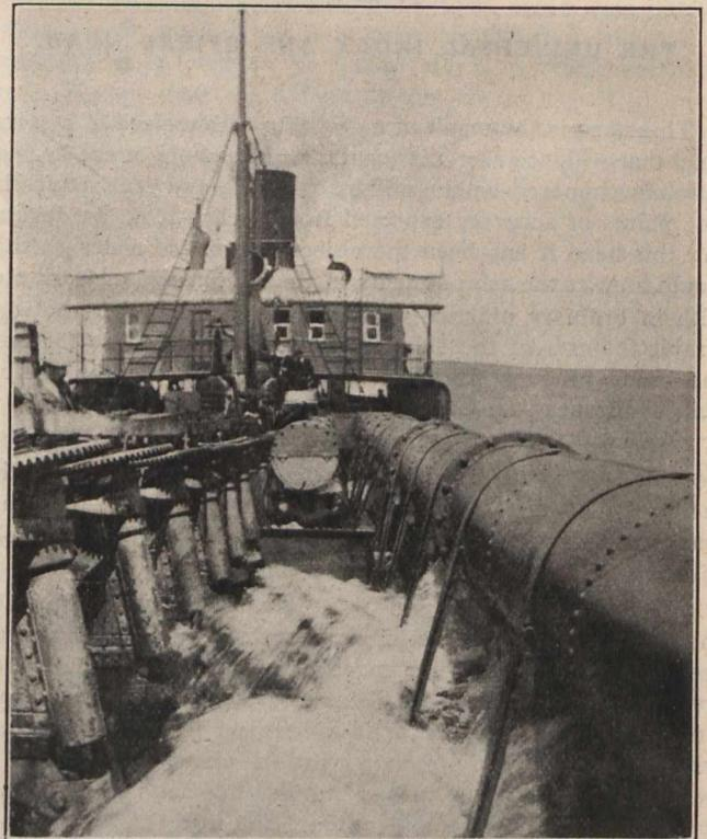
Fig. 1.—The "Calveston," looking aft, showing water pouring from openings in long pipe into hoppers... The gearing operates the hopper doors.
