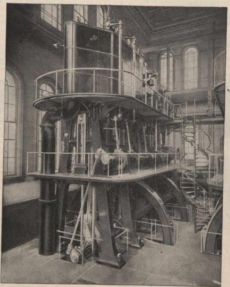
Allis-Chalmers Vertical Triple-Expansion Pumping Engine.
