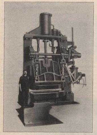
Fig. 4. The Drawing Press.
