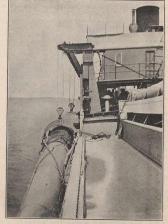
Fig. 4.-Suction Pipe partly submerged, showing teather joint.
