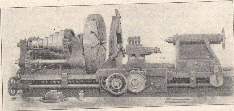
form and wide enough to prevent the tool over-hanging the front when turning full swing on the lathe. This lathe is designed for use of modern high-power tool steels and is an especially powerful machine.
