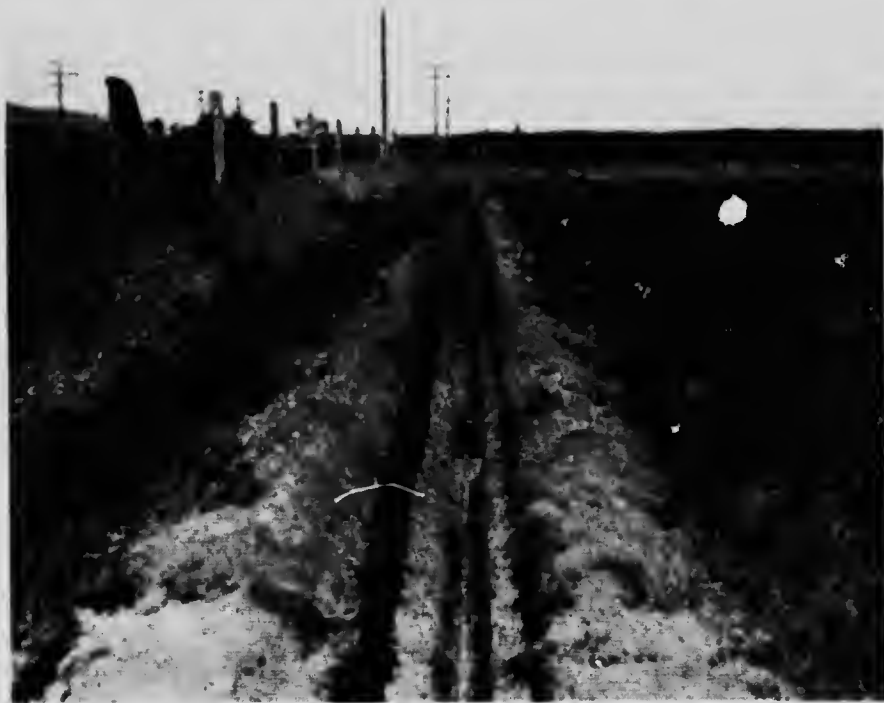
FIG. 16.—Ditch near Sussex, N. B., dug by traction ditcher. (Original).
