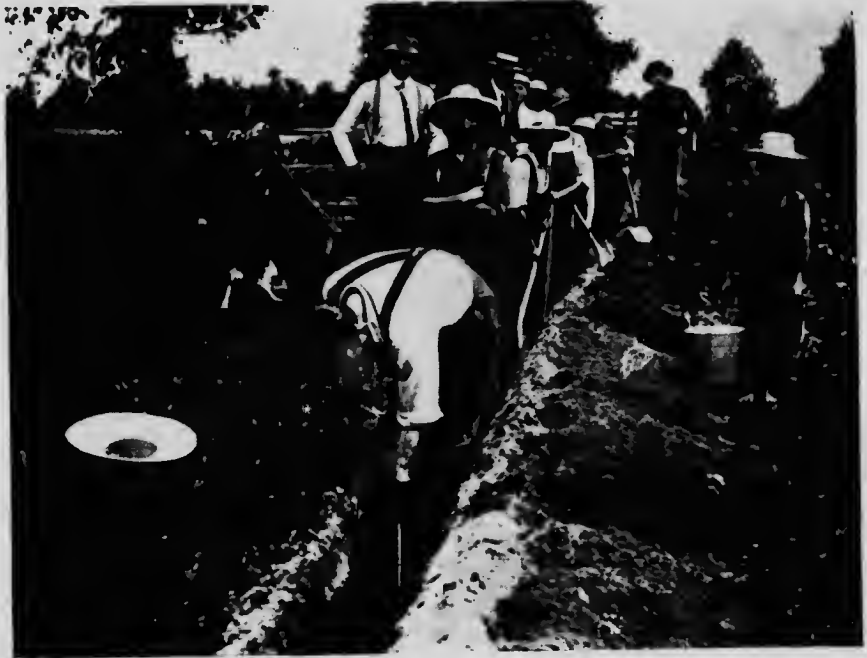
FIG. 12.—Digging trench at Burford, Ont. This shows the spirit of co-operation which was so apparent among the farmers. (Original).
