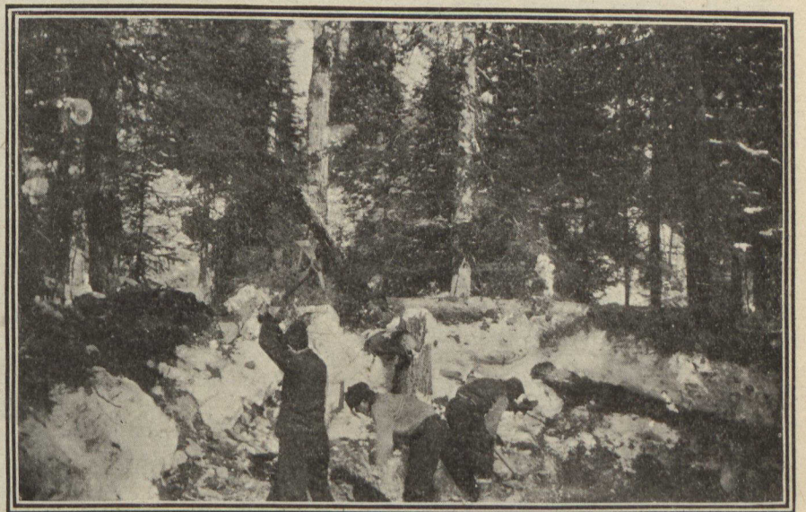
These Dagoes are not digging Gold; but excavating for a Residence.
