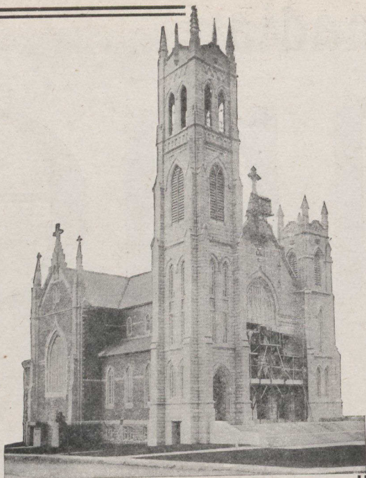
St. Viateur R.C. Church, Montreal, Roofed with ASBESTOSLATE
