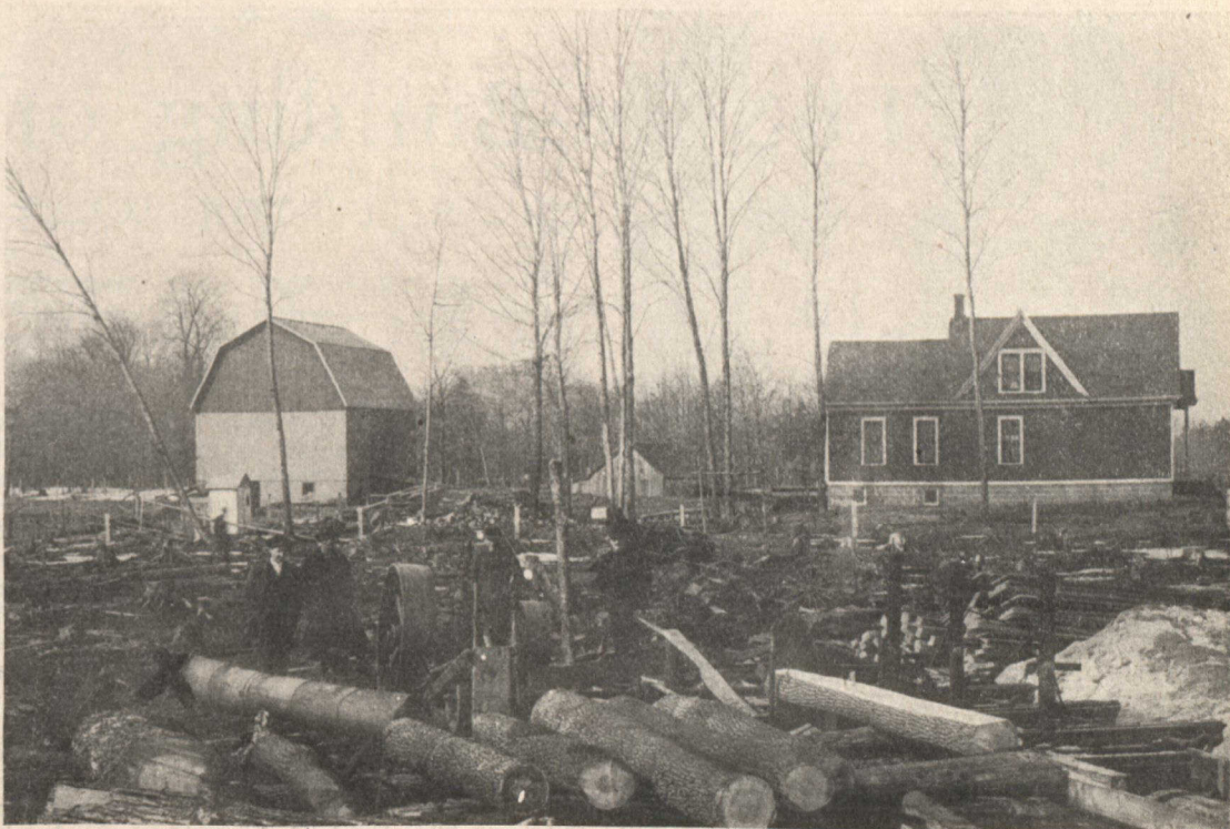
Mill-yard in Lambton County where the Explosion took place. Cross shows the spot where the Boiler used to be
