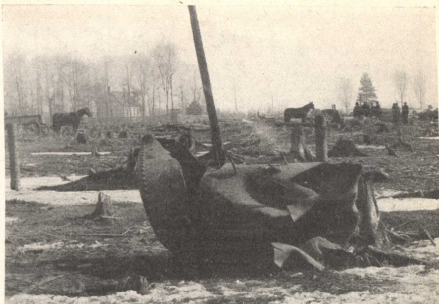
Fire-box of Saw-mill Boiler hurled 300 feet and stopped by a tree
