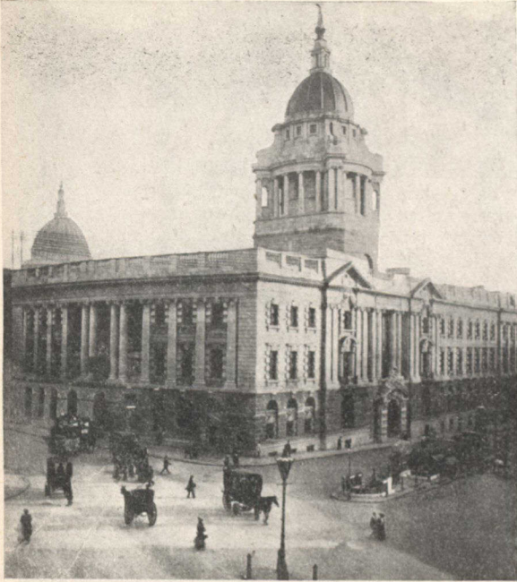
The New Central Criminal Court, known as the "New Bailey."
