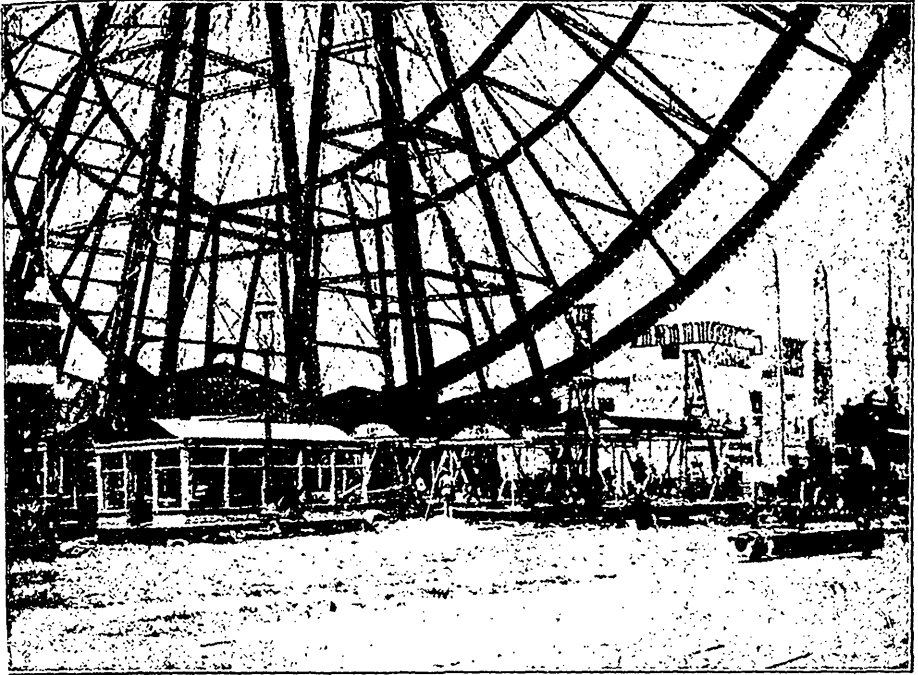
VIEW SHOWING THE LOWER CONSTRUCTION OF THE FERRIS WHEEL.
