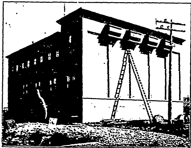
SUBSTATION AT FORT WILLIAM, HIGH TENSION END.
