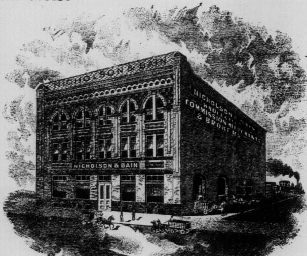
BANNATYNE ST. EAST. TRANSFER TRACK.
