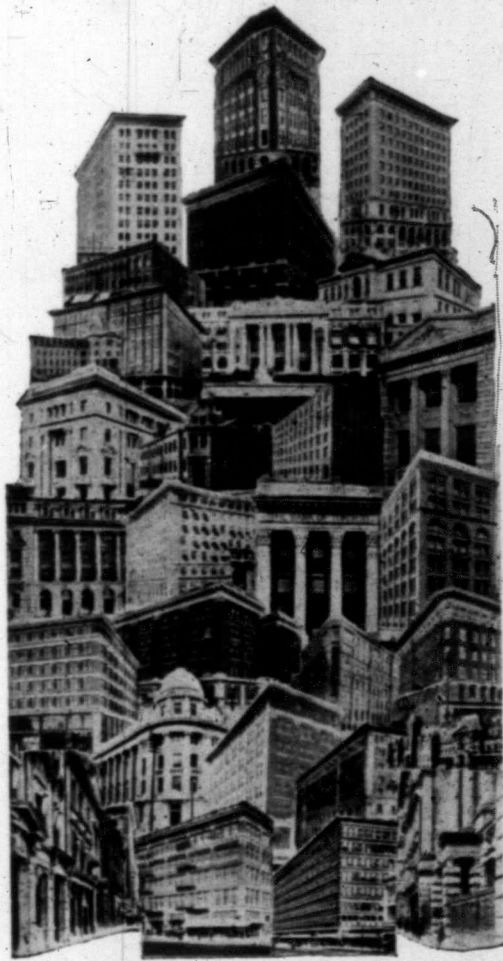
The Corner Posts of the Convention City.
