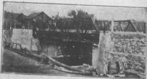
The New "Robertson's Bridge" at Clydeville.
