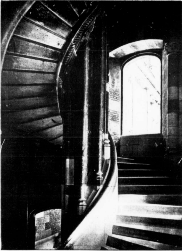
FIG. 28.—Staircase in the old wing of the Château of Blois ; showing single right-handed spiral
