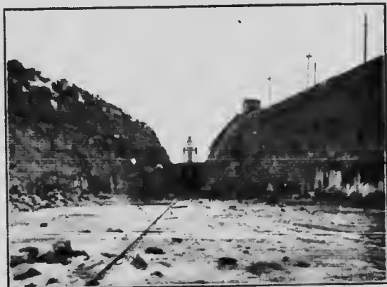
FIG. 8—VIEW UP CANAL FROM FLOOR OF FOREBAY
