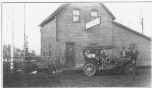
Dominion Land Office, Grouard
