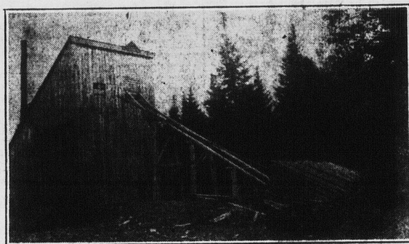
SAMPLE OF STRUCTURE AT BANK HEAD. THIS IS THE BUILDING ERECTED AT NO. 6 SHAFT.
