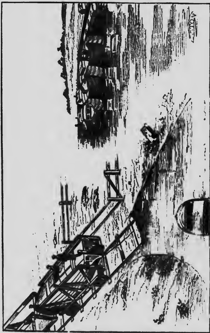
ALLEGHENY PORTAGE RAILWAY Canal boat ascending an inclined plane
