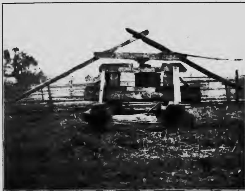
HORSE-POWER CRUSHER—EARLY SUGAR MILL
