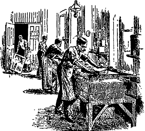
PREPARING THE STONES.
