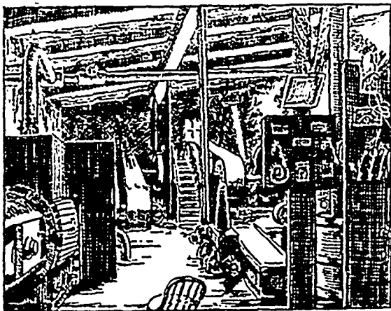
A BIT OF THE POWER HOUSE, KINGSTON.
