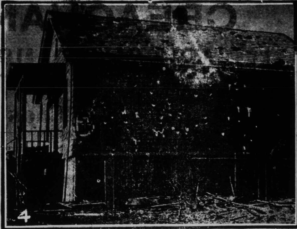
This picture shows vividly the effects of exploding shells as a result of the great explosion and fire which wrecked the Canadian Car and Foundry Company at Kingsland, N. J. The house, through which scores of projectiles passed, is located one mile from the scene of the disaster.
