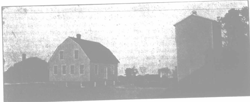
Canning Factory and Cold Storage. New Administration Building in Background.
