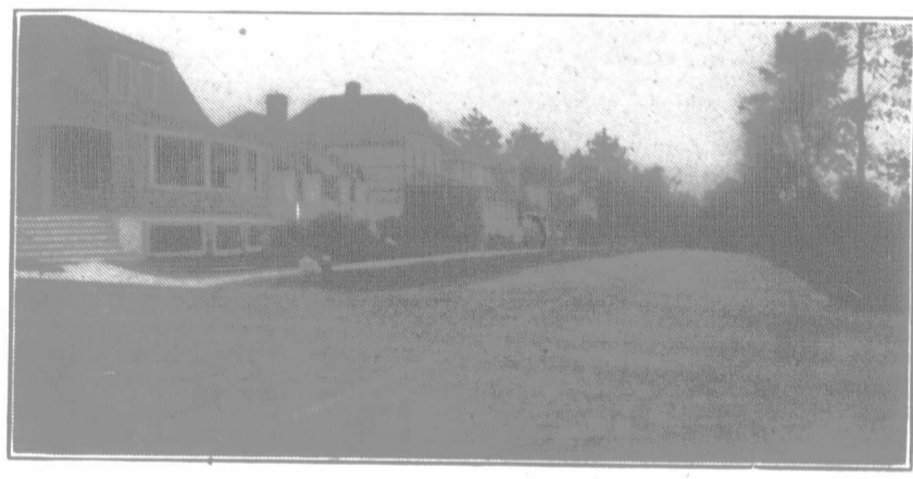
Roadway in Grand Mere, Province of Quebec, constructed with "Tarvia-X" in 1912.
