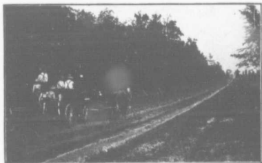
A ROAD GRADER AT WORK
