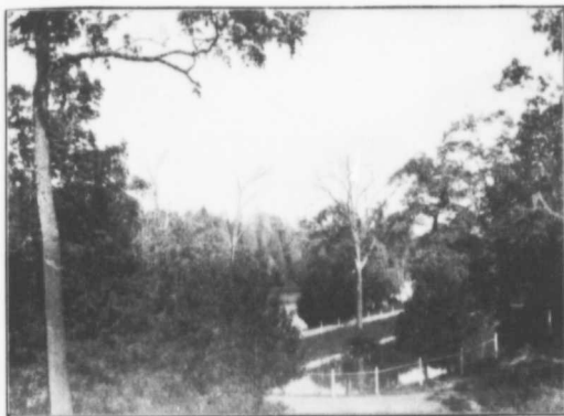
ALONG THE RIVERSIDE, NEAR THE PUMP-HOUSE.
