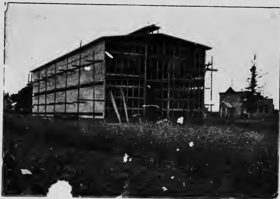
Tobacco curing barn in course of erection
