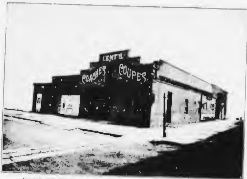
BARN OF SEYMOUR FINNEY, ESQ., DETROIT, MICHIGAN. A shelter for fugitives in Detroit, formerly standing where the Chamber of Commerce Building now stands.
