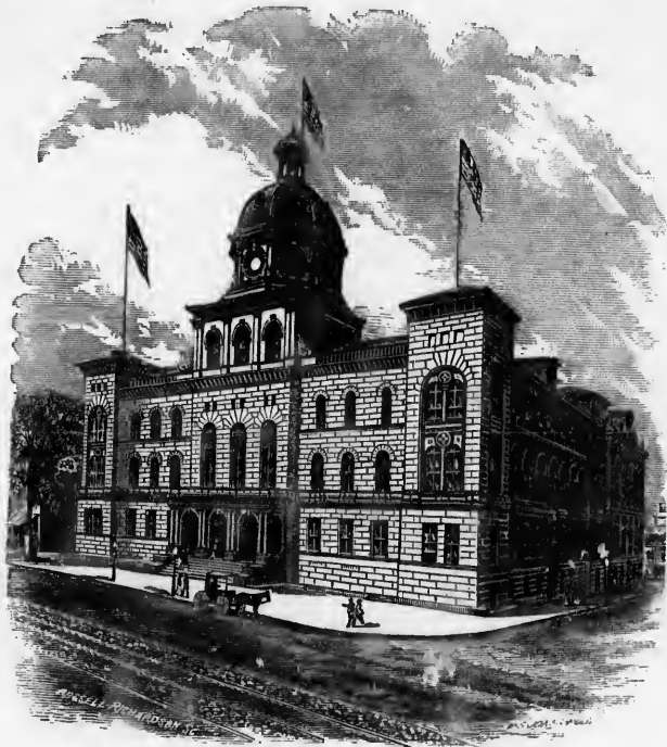
CITY HALL, PORTLAND.
