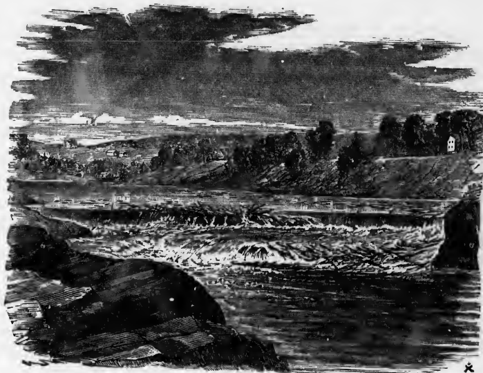
NORTH CHANNEL DAM, AT SKOWHEGAN, ME.
