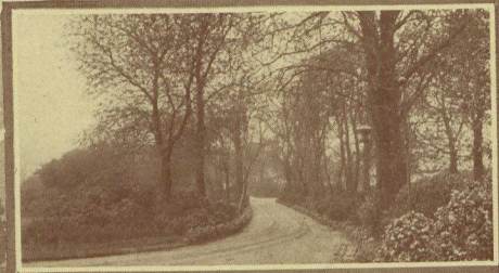
ENTRANCE DRIVE TO KINGSWOOD
