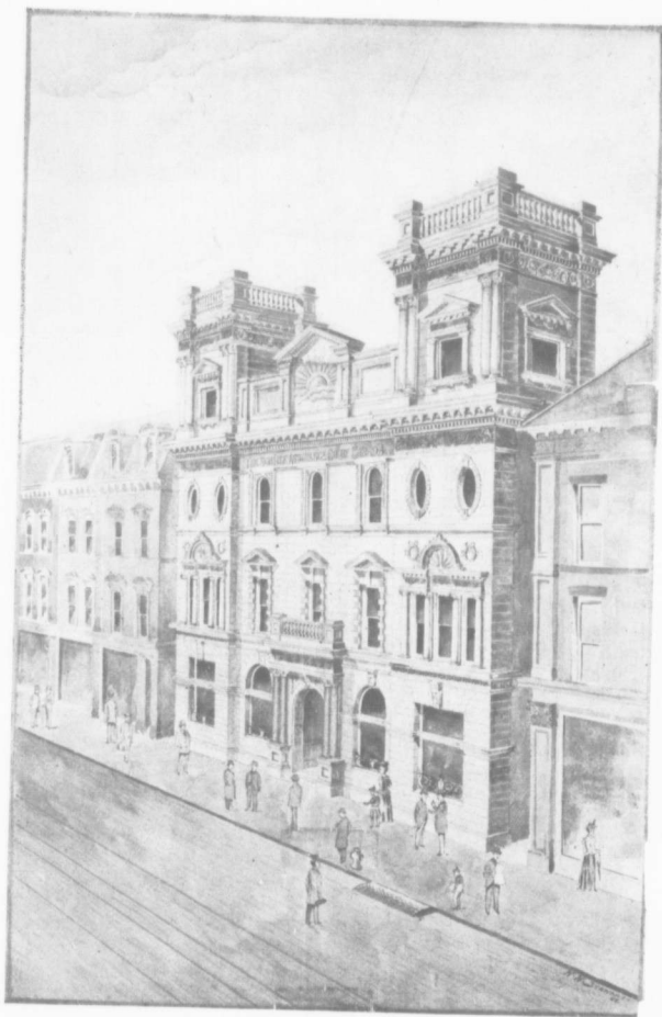
THE NEW BUILDING OF THE SUN LIFE ASSURANCE COMPANY OF CANADA, AT HAMILTON, ONT.
