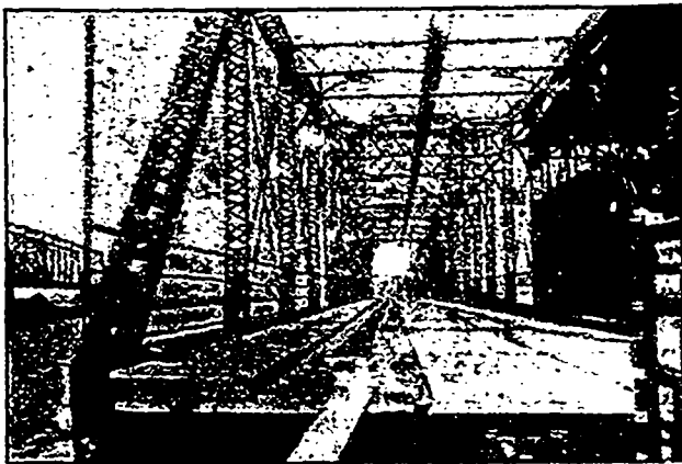
BURLINGTON CANAL BRIDGE LOOKING EAST, WITH G.T.R. BRIDGE ON LEFT.
