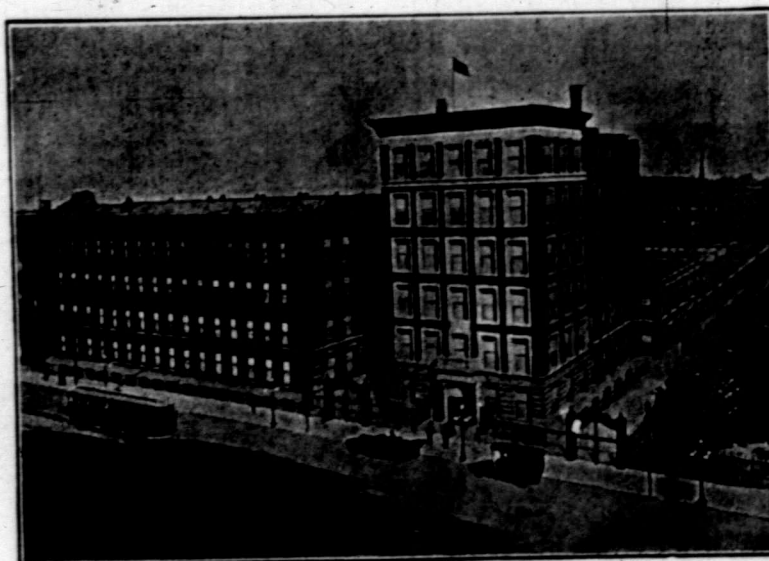
FIRE PROOF BUILDINGS
