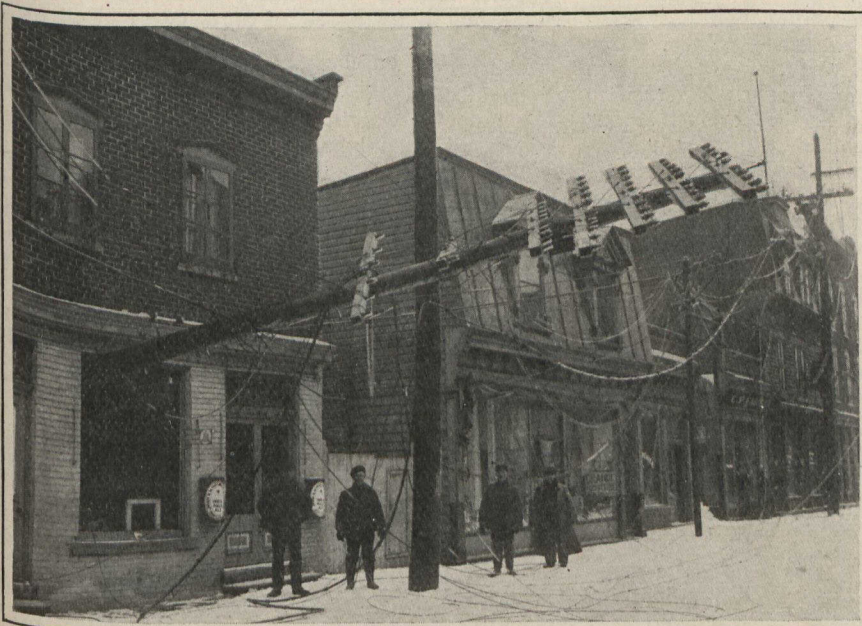
Montreal—This pole was broken near the ground and then swung through the plate glass window of a saloon.
