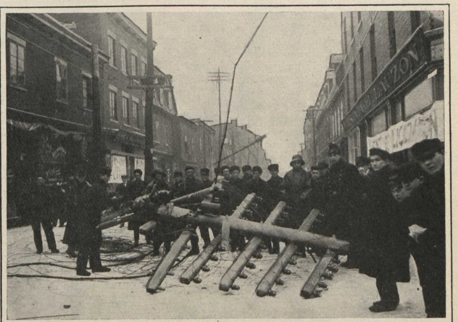
Montreal—The Ice on the wires was heavy enough to bring down telegraph and telephone poles as occurred once in Toronto some years ago.
