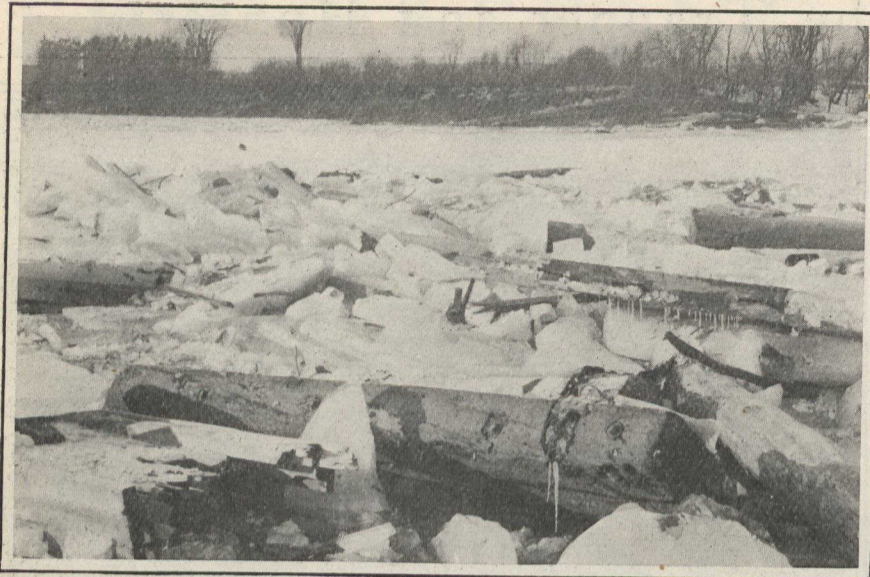
A view of the wreckage, showing a five-timber boom snapped off short.
