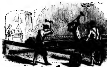
RIVETING A COLUMN.
