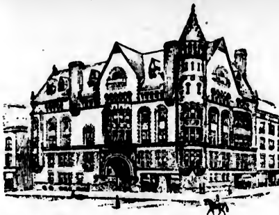
NEW Y.M.C.A. BUILDING, In course of erection on Dominion Square.
