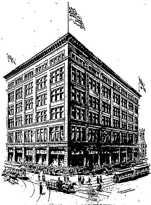
MAIN BUILDING, CORNER YONGE AND QUEEN STREETS
