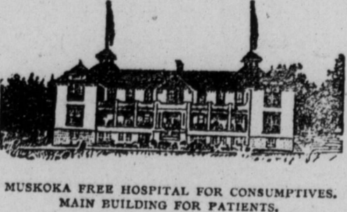
MUSKOKA FREE HOSPITAL FOR CONSUMPTIVES. MAIN BUILDING FOR PATIENTS.
