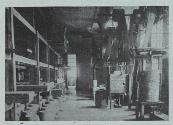
Pugging Machine, showing orifice and cutting-board in foreground. Crucibles are drying on racks preparatory to firing.
