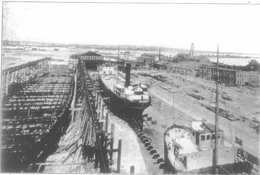
Western Dry Dock and Shipbuilding Company's plant at Port Arthur where the W. Grant Morden, the largest freighter ever built in Canada, was launched a few days ago.
